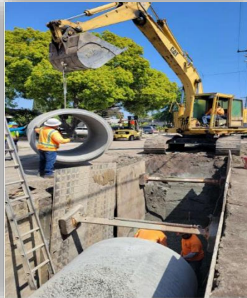
The Acacia-Josephine Storm Drain in construction.
