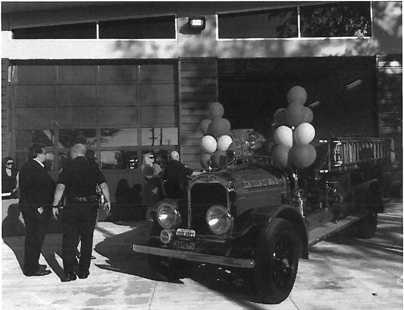
A FIRE ENGINE from the original Garden Grove fire service in the 1920s contrasts with the brand new Station 6 on West Street at Tuesday's dedication (Orange County Tribune photo).
