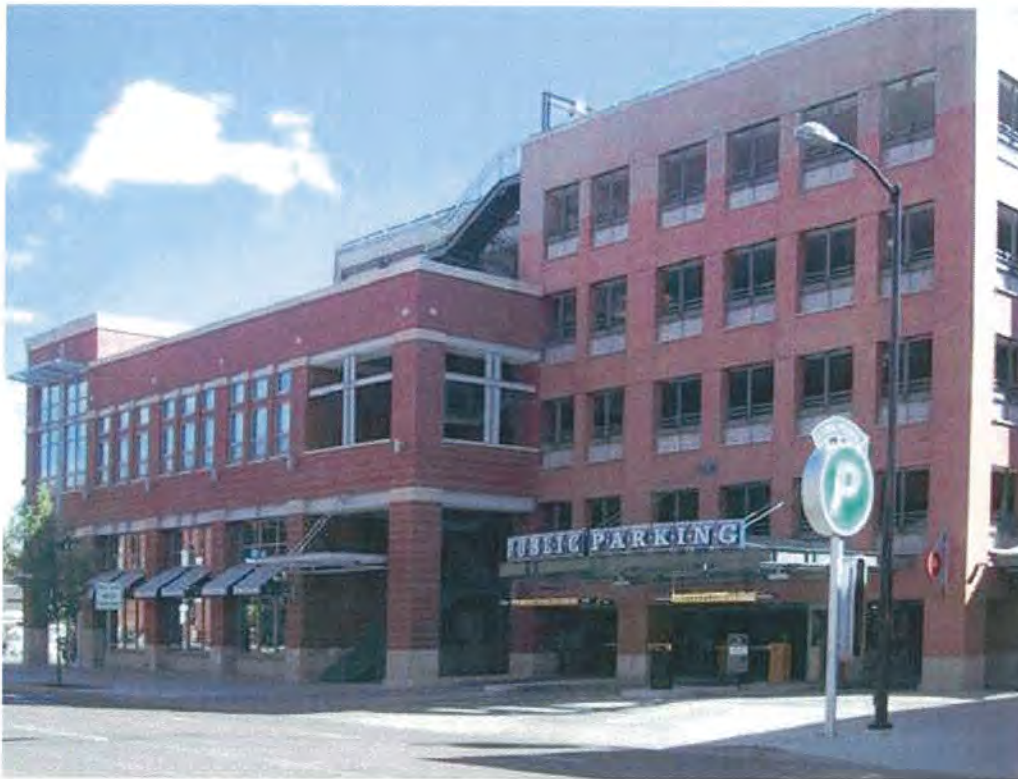
Photo 9.18-9: Example of Parking Structure Architectural Treatment
