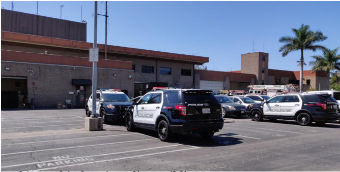
Parking Behind Main Police Building
