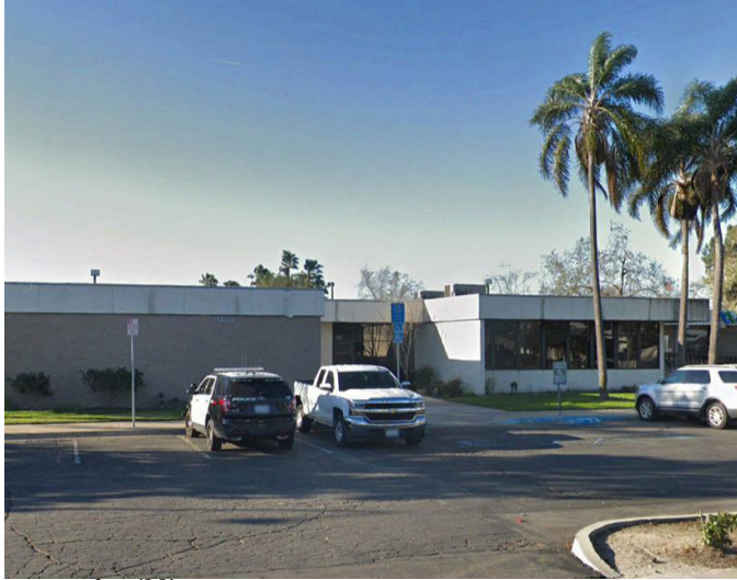
Front of Building
