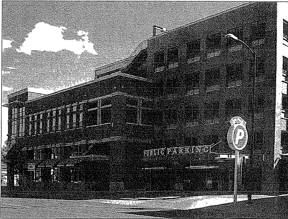
Photo 9.18-9: Example of Parking Structure Architectural Treatment
