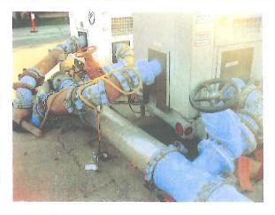
notify the Contractor and the District in the event of failure of any bypass system that could result in a spill. Noise should be mitigated in residential and business areas since the pumping may exceed the noise ordinance limitations. An example of a sound attenuated bypass pump is provided as **Figure A-2** in **Appendix A**.
