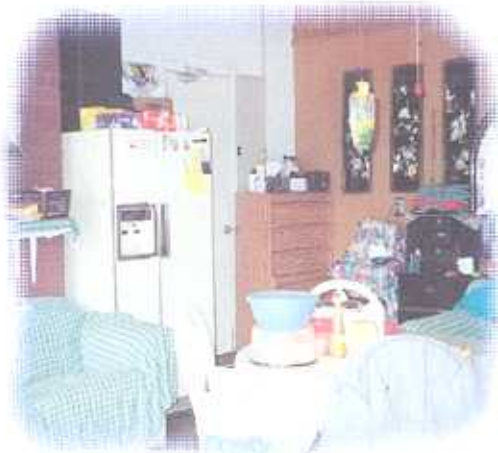
Garage illegally converted to living Quarters.
