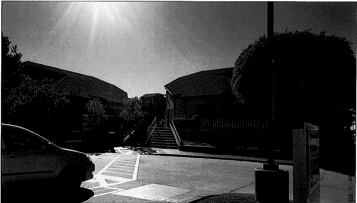
View of the general office uses to the west facing west.
