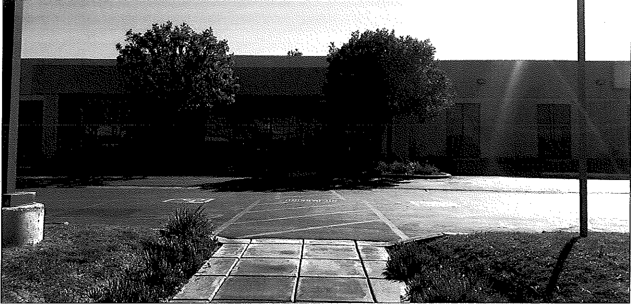
View of the existing building.
