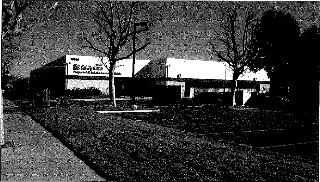
View of the CalOptima located to the east facing east.
