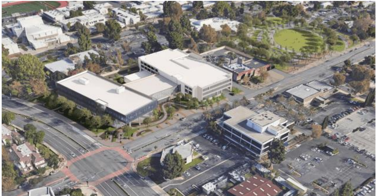
A BIRD'S EYE view of the planned Civic Center Revitalization project (City of Garden Grove).
