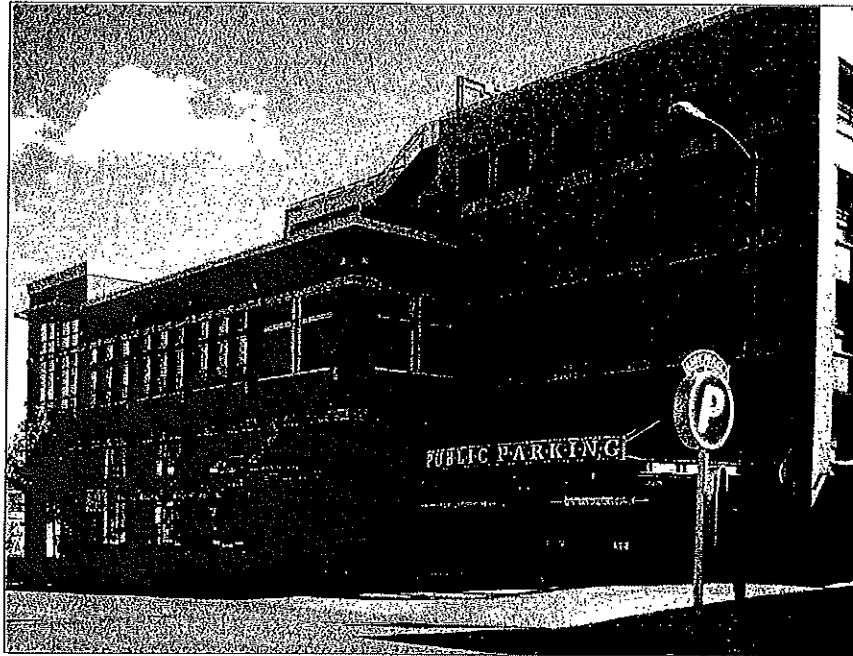
Photo 9.18-9: Example of Parking Structure Architectural Treatment
