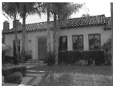
A Spanish Revival office in Placentia
